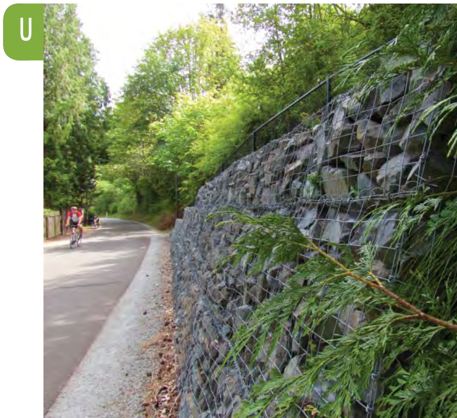
Figure 4U: Example of Gabion Retaining Wall
