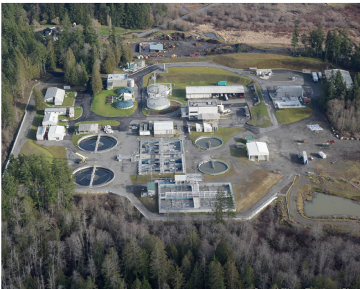
Aerial view of Central Kitsap Treatment Plant
