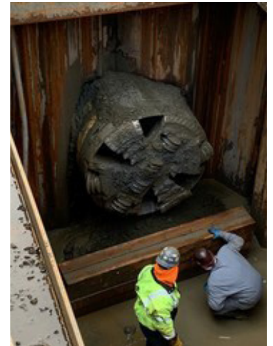
Drill head of the micro tunneling machine entering the receiving pit
