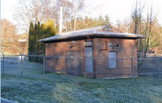
Pump Station 19 near Nels Nelson and Bucklin Hill Road will be upgraded this summer
