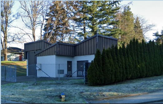
Pump Station 4 in Silverdale is being upgraded for capacity
