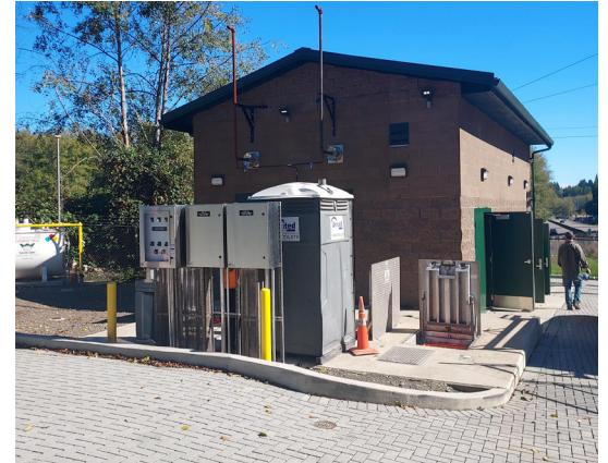
New Pump Station 19 building on Bucklin Hill Rd. adjacent to Waaga Way
