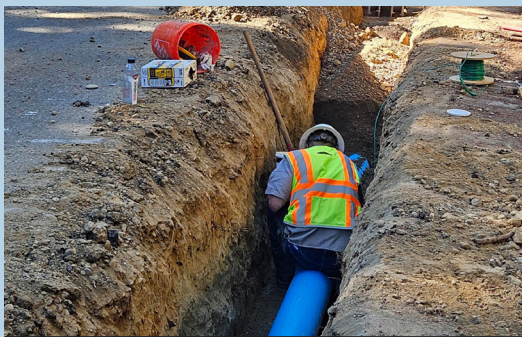
Sewer Utility crews repaired forcemain in East Bremerton
