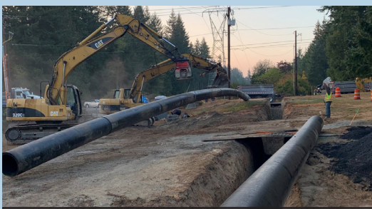
Bangor/Keyport Forcemain Replacement project replaced 5 miles of forcemain
