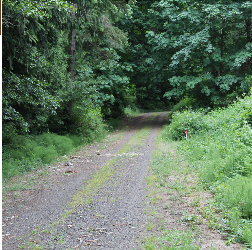
Figure 2W: Road Type 3 - Narrow, Gravel, Frequent Use
