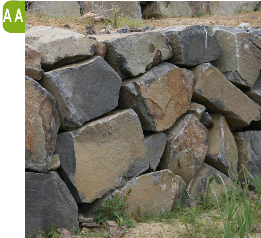
Figure AA: Example of Rockery Retaining Wall
