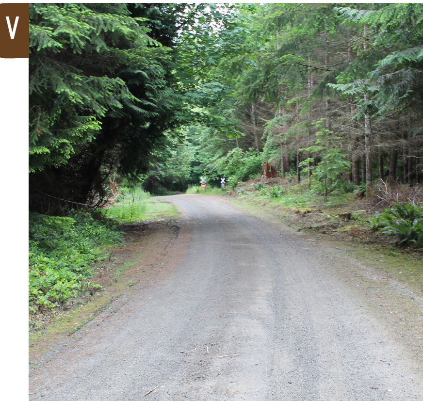
Figure 2V: Road Type 2 - Wide, Gravel, Frequent Use
