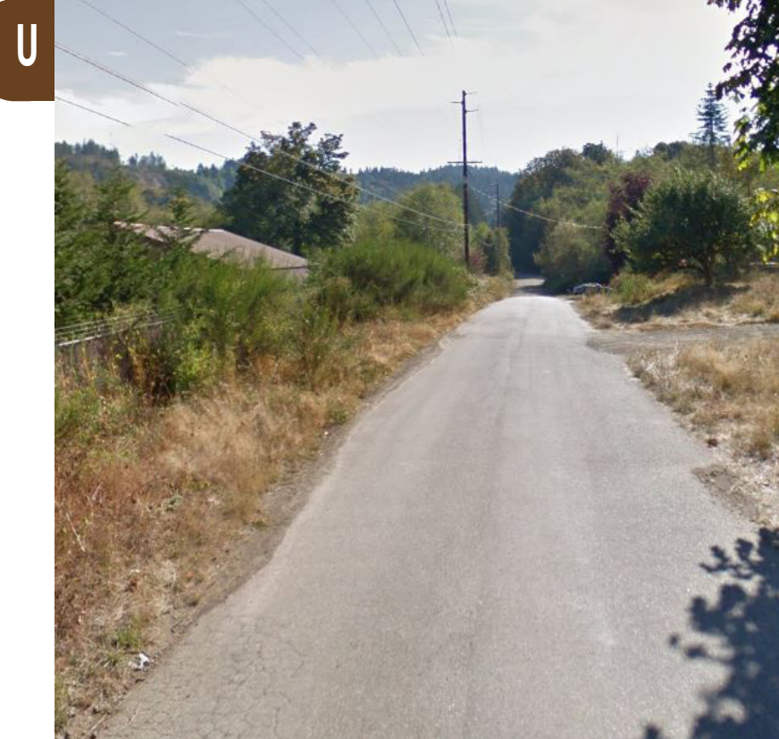
Figure 2U: Road Type 1 - Narrow, Paved, No Striping
