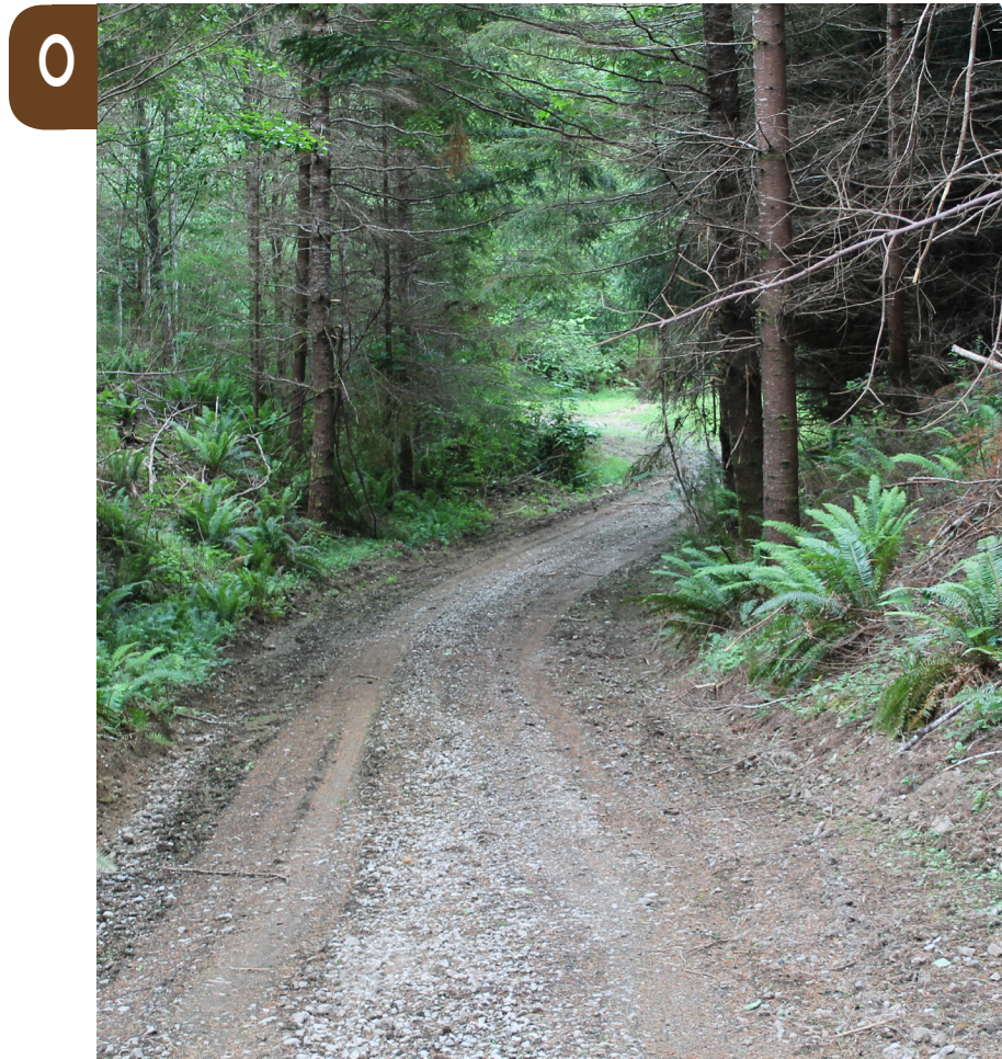
Figure 20: Road Type 4 With a Slope Greater Than 8%
