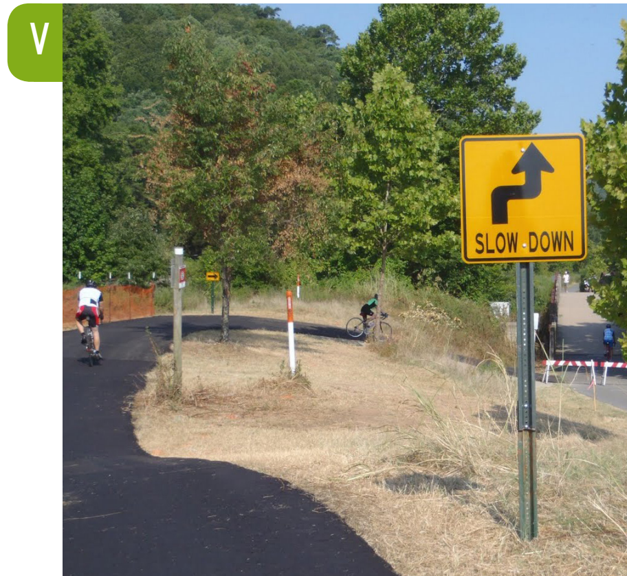
Figure 3V: Typical Regulatory Sign Along Trail
