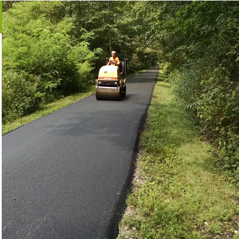
Figure 3AC: Paved Trail Construction
