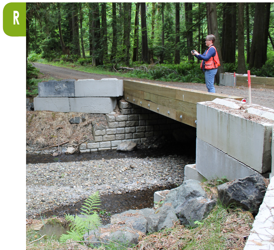
Figure 3R: Nearby Bridge
